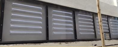
Louvers can be installed at any height of sheds promtly, which also allows natural fresh air to pass through along with natural daylight in to the spaces at any height.
