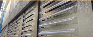
Compare to metal Louvers these are light in weight and can be installed easily without any hassle during installation.
