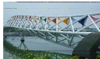
Atal Bridge - Ahmedabad
