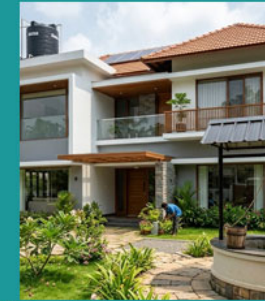
Well & Overhead tanks
